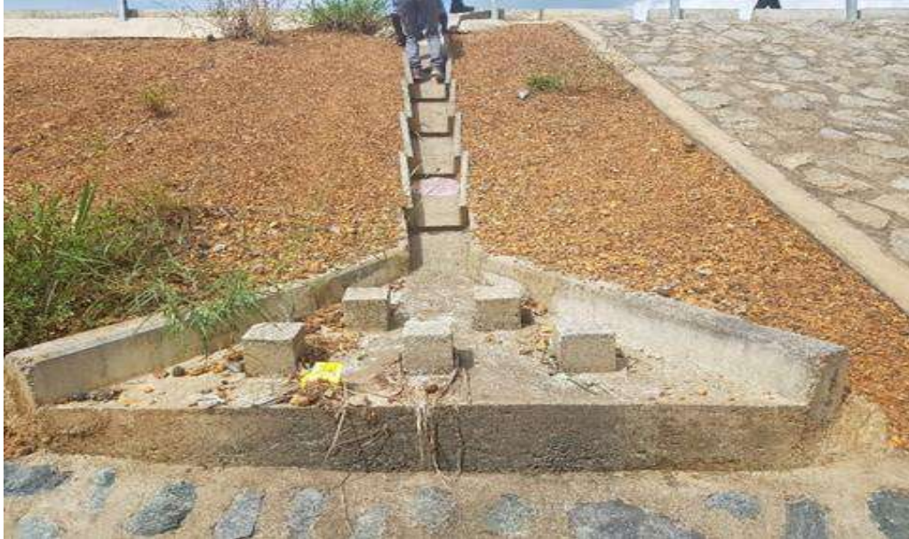
Figure 20: Typical down chute
