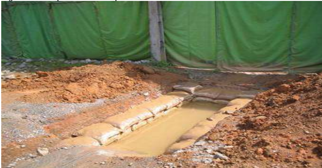
Figure 64: Sample silt removal ponds
