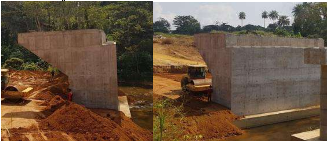
Figure 16: Cantilever solid wall abutment
