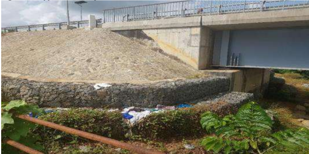
Figure 18: Typical erosion protection at Abutment
