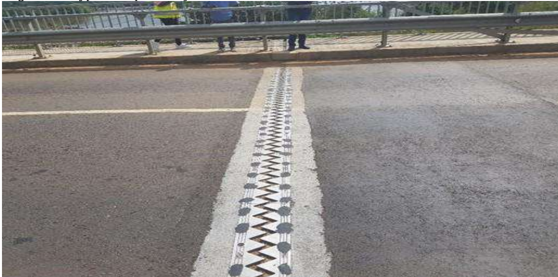
Figure 17: Typical Expansion joint
