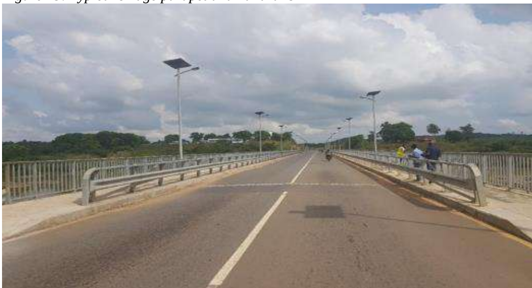
Figure 19: Typical bridge parapet and handrails
