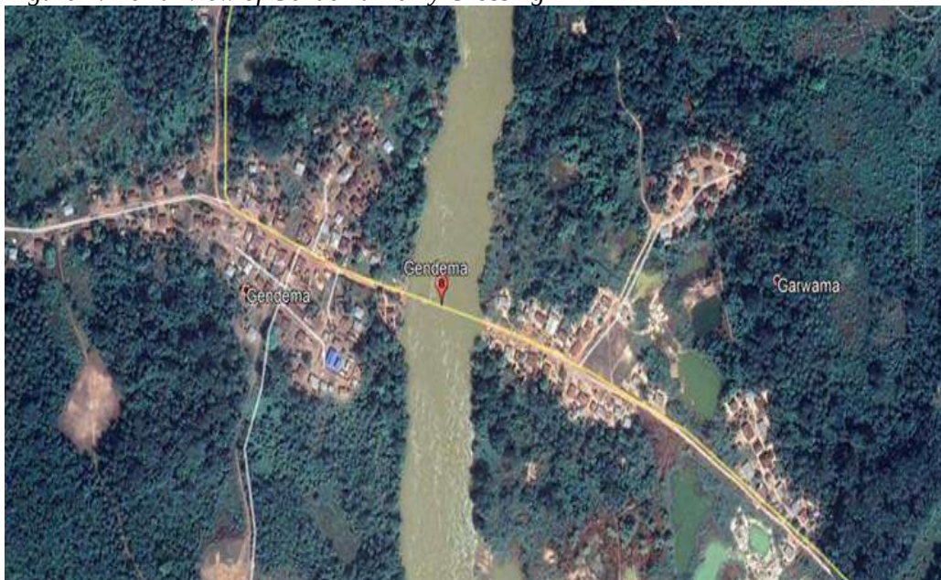
Figure 7: Aerial view of Gendema Ferry Crossing
