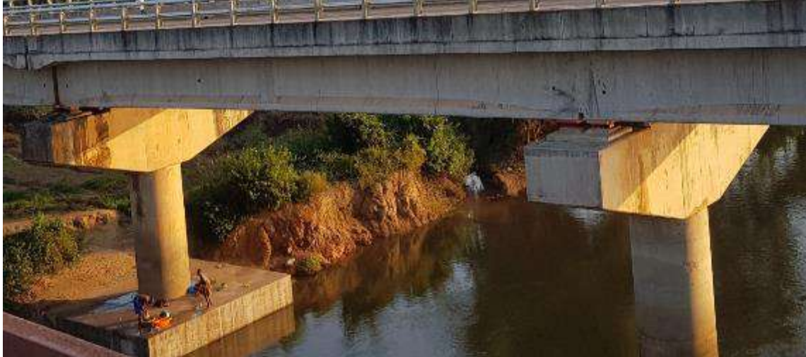
Figure 15: Single column with hammerhead Pier
