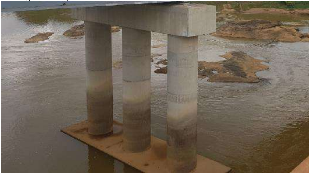
Figure 14: Typical Multiple Circular Columns Pier
